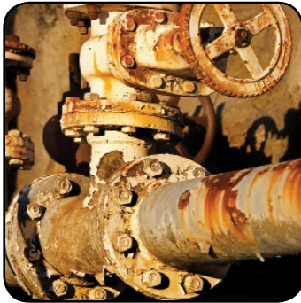
Flange Corrosion
